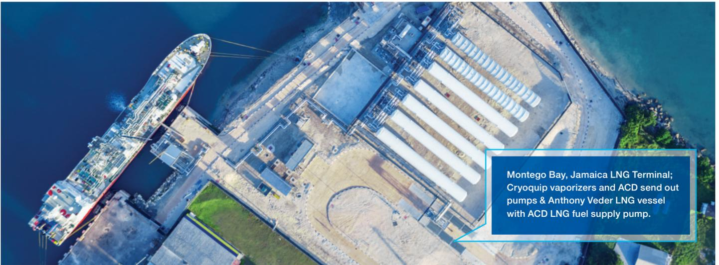
Montego Bay, Jamaica LNG Terminal; Cryoquip vaporizers and ACD send out pumps & Anthony Veder LNG vessel with ACD LNG fuel supply pump.
