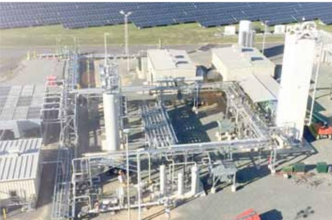
60,000 gpd installation with heavy hydrocarbon removal system.
