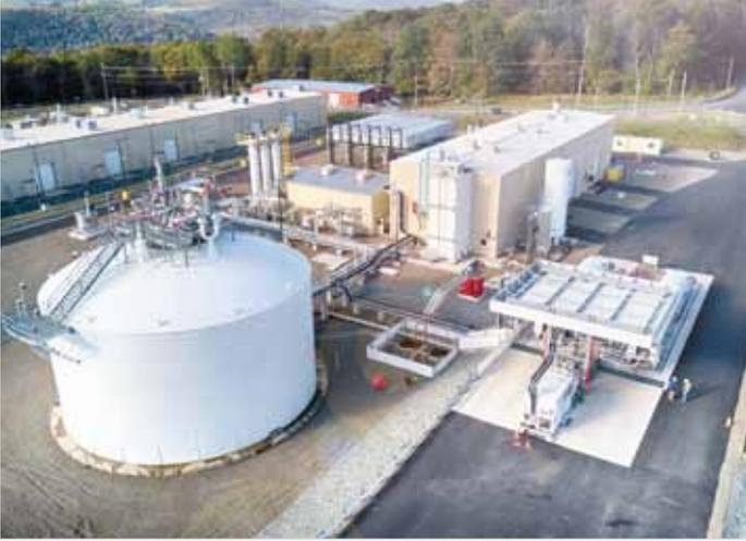
150,000 gpd installation. Gas Turbine driven Refrigerant Compressor.
