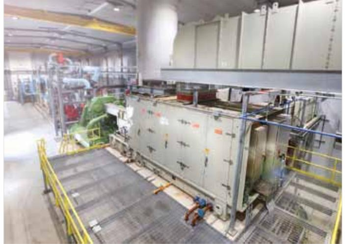
Gas Turbine driven Refrigerant Compressor.
