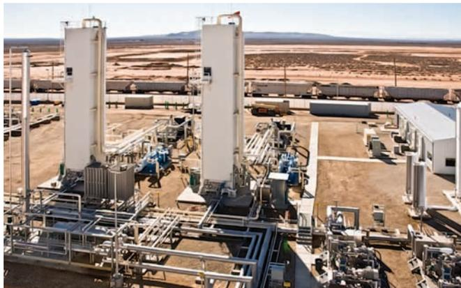
FIG. 9. An LNG plant with multiple trains. Photo courtesy of Clean Energy Fuels.
