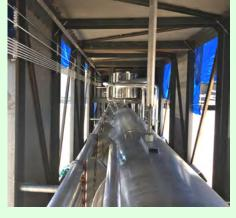
COLD BOX SHIPPED PRE-FABRICATED AND INSULATED WITH PERLITE, NO FIELD ACCESS
