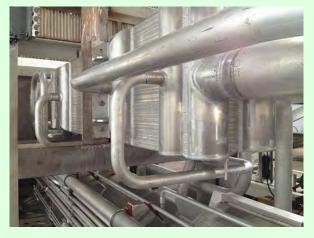
BRAZED AL HEAT EXCHANGER AND PIPING
