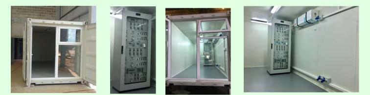
SHIPABLE ISO CONTAINER CONTROL ROOM AIR CONDITIONING AND INSTALLED ANALYSERS WITH LIGHTING, POWER, SOUND PROOF DOORS AND CLADDING
