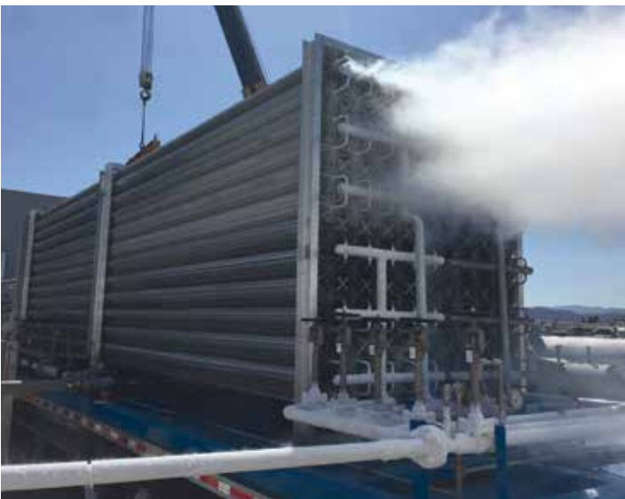
Figure 5 – Horizontal fan ambient in operation
