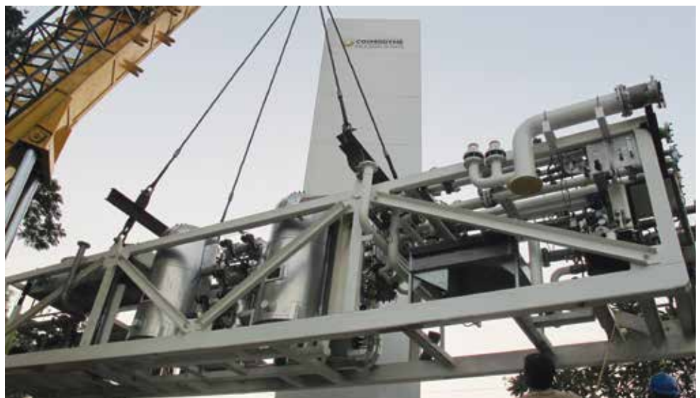
Spruce complete warm end being installed
