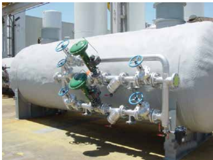
Dual Steam Control Valves
