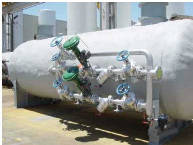
Dual Steam Control Valves
