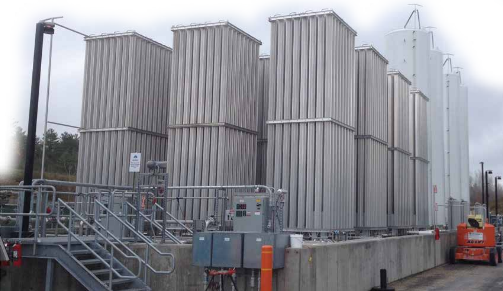
Figure 4. Satellite LNG ambientvaporizer system for industrial heat and power in the Northeastern U.S.
