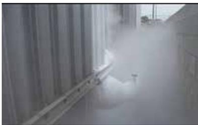
One of the most important aspects when installing ambient vaporizers is to make sure the fog and cold air downdraft being created has the clearance to properly disperse and dissipate to allow new warm air into the vaporizer array. This is done by having the proper clearance from the ground and other surrounding objects. Walls, tanks, and other vaporizers
