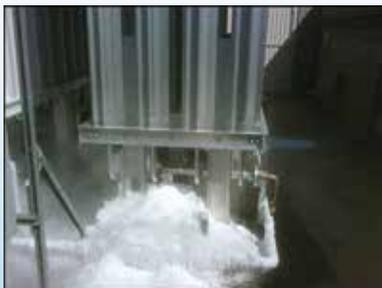
The location of an uninsulated liquid line that feeds the vaporizers is very important, and improper installation can result in unnecessary problems. The liquid line should not be installed directly underneath or too
