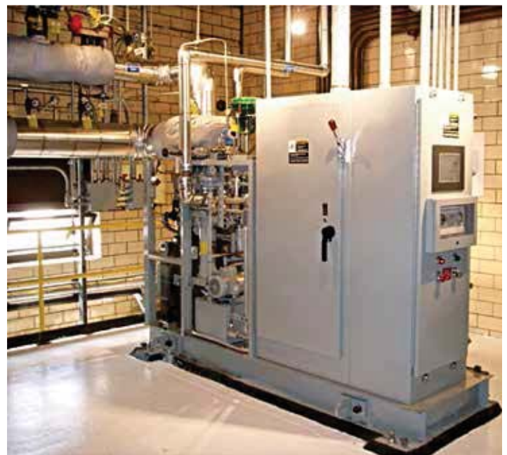
Figure 4 – Microsteam Power System 275 kW installed at Con Edison Steam Station NYC
