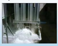
The location of an uninsulated liquid line that feeds the vaporizers is very important, and improper installation can result in unnecessary problems. The liquid line should not be installed directly underneath or too
