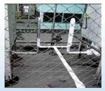
ambient vaporizer naturally begins to build up ice as it's running, decreasing its performance over time. Continuous flows require switching to an idle vaporizer to maintain the proper discharge temperatures. There are two different
