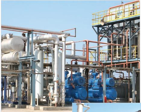
scope of supply included a purification, compression, dehydration, liquefaction, and stripping system, 2x250 metric tons (MT) of bulk CO<sub>2</sub> storage, and five mobile CO<sub>2</sub> transport trucks. In addition to the CO<sub>2</sub> processing equipment, the system included a motor control center, PLC control system with SCADA (Supervisory Control and Data Acquisition), an ammonia refrigeration system, field piping, wiring, and insulation.
