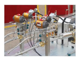
With the integration of a Programmable Logic Controller (PLC), the unique pumping system is able to automatically start, stop, and switch pumps. The Short Message Service (SMS) text-enabled skid allows the client to monitor the system remotely—a significant advantage for un-manned pumping installations required at remote customer sites.
