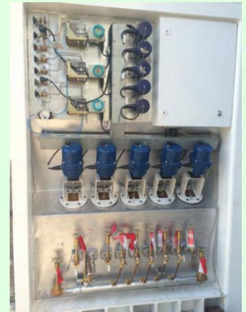
CANNED CRYOGENIC VALVES
