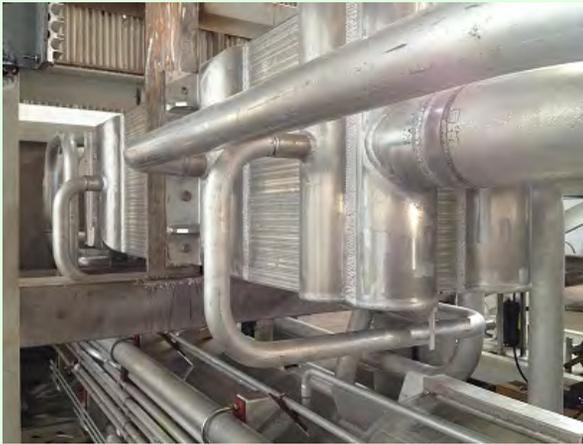
BRAZED AL HEAT EXCHANGER AND PIPING
