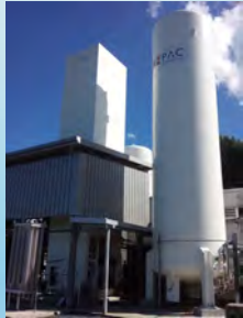
PREFABRICATED AND CONTAINER SHIPABLE BUILDING DESIGNED FOR PLANT
