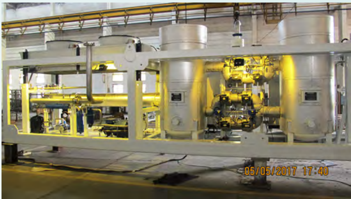
TSA DRYER CONTROL VALVES lighting included pre-installed on all skids-
