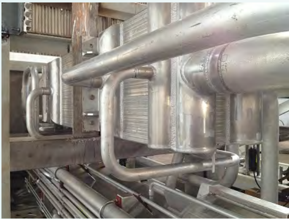
BRAZED AL HEAT EXCHANGER AND PIPING
