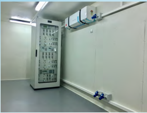
SHIPABLE ISO CONTAINER CONTROL ROOM AIR CONDITIONING AND INSTALLED ANALYSERS WITH LIGHTING, POWER, SOUND PROOF DOORS AND CLADDING
