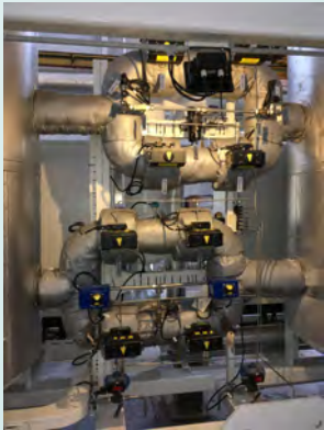
ADSORBER BED VALVES WITH SOFT INSULATION
