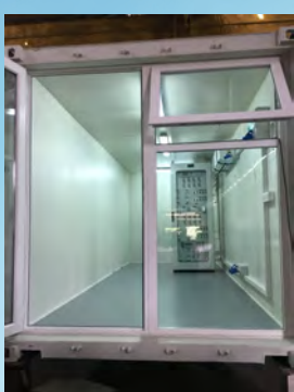
SHIPABLE ISO CONTAINER CONTROL ROOM AIR CONDITIONING AND INSTALLED ANALYSERS WITH LIGHTING, POWER, SOUND PROOF DOORS AND CLADDING
